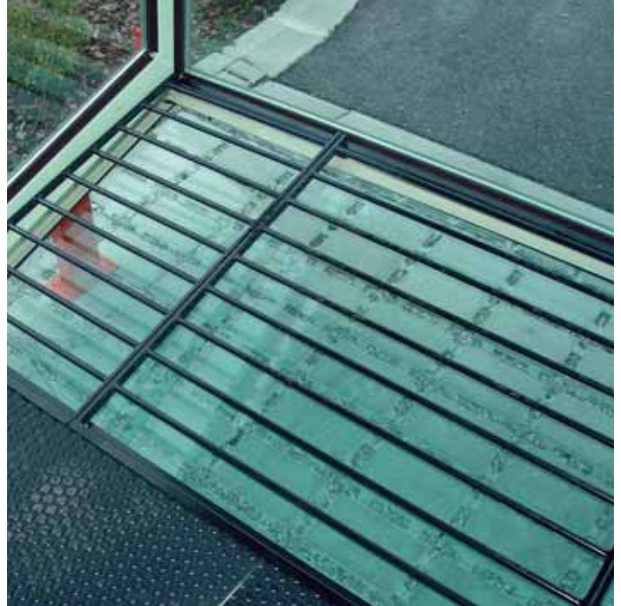
GS03 Walkable safety floor glasses, 40 mm thick, complete with footrest grids
