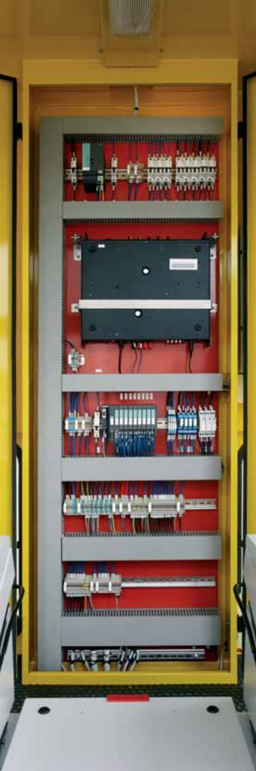
XT01 Supply and wiring of electrical panels complete with electrical material
