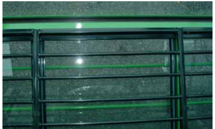
GS05 Floor glasses, 3+3 mm thick, mounted on removable frames with interior and exterior safety grids
